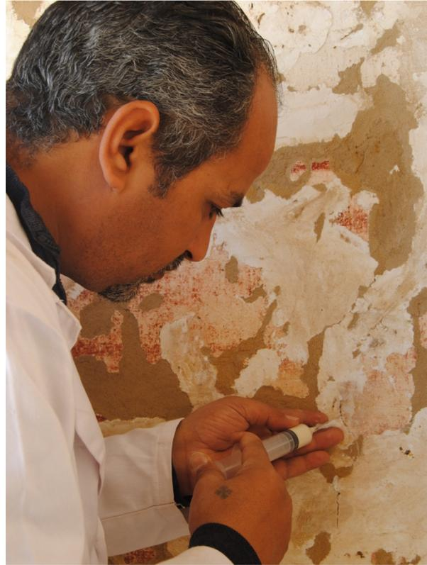
Fig. 12: Field school 2018- Application of plaster renderings with conservation mortar in GB10 (M3/SS). Thin green tubes have been included for later grout injections. Fig. 13: GB 24 (M09/SE), grouting of smaller hollow areas within painted plaster surfaces was done directly with syringes and cannulas.
