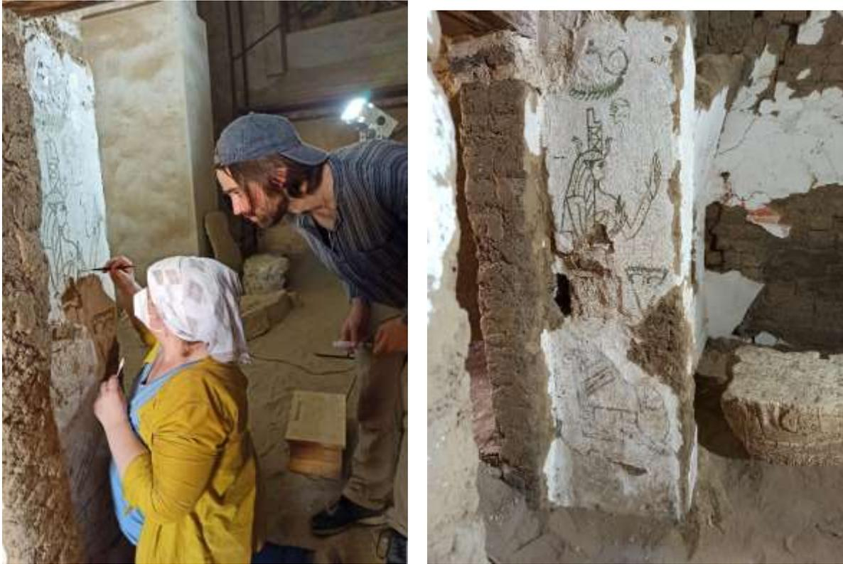
Main room, during (left) and after conservation (right): consolidation of paint layer, rendering plaster edges and grouting were the appropriate measures carried out
