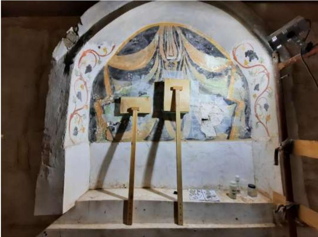
Support system set up before grouting
