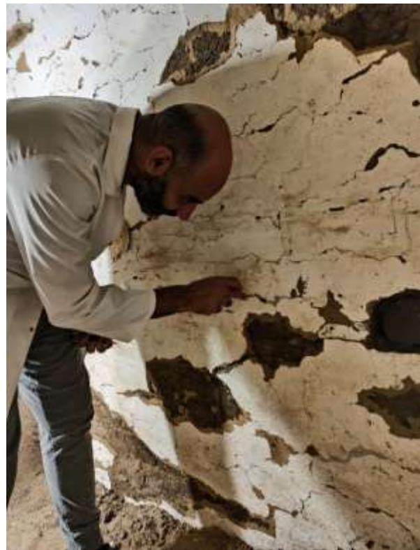
Securing mud plaster by rendering the edges, western walls on ground floor
