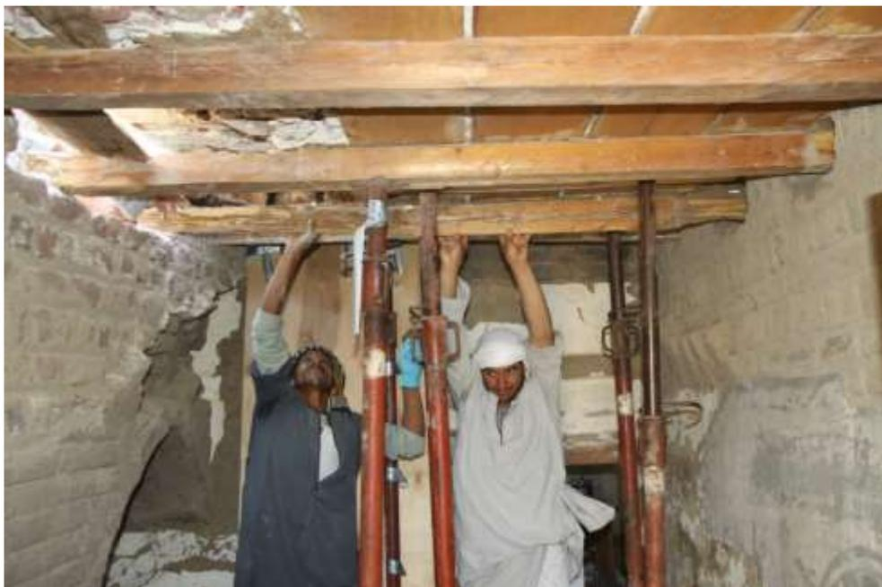
Taking out rotten beams in the antechamber by sliding them sideways (2019)
