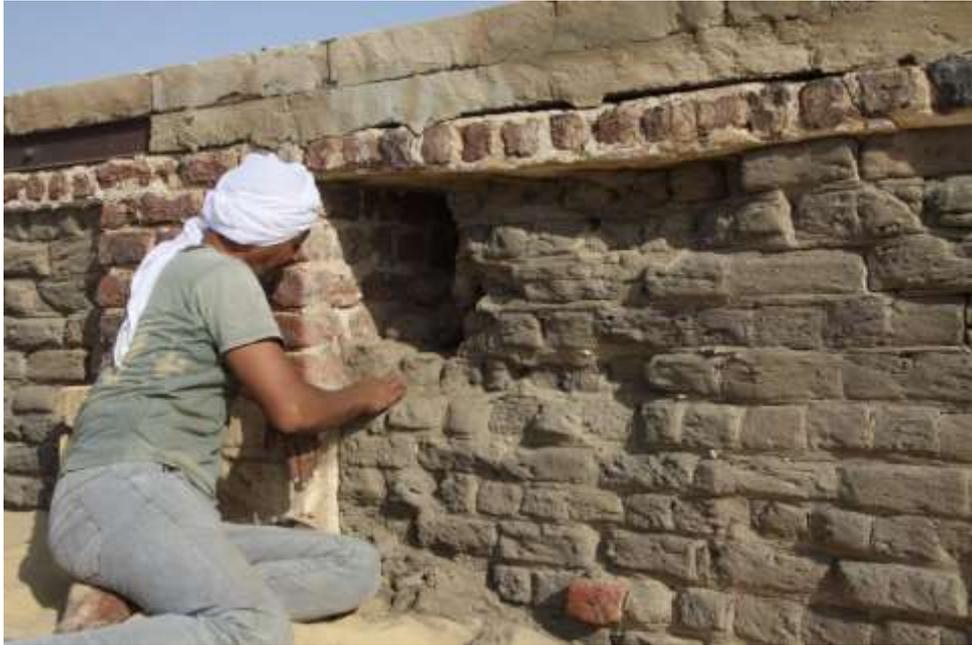
Repairing the ancient mud brick masonry under the roof from the 1930s (2019)
