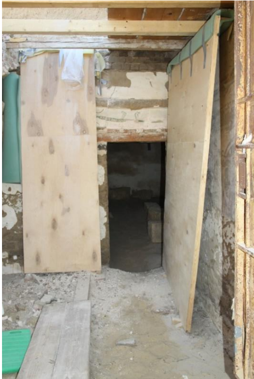
Antechamber (GB33A) (left) and GB33B (right) with protective shields during roof work
