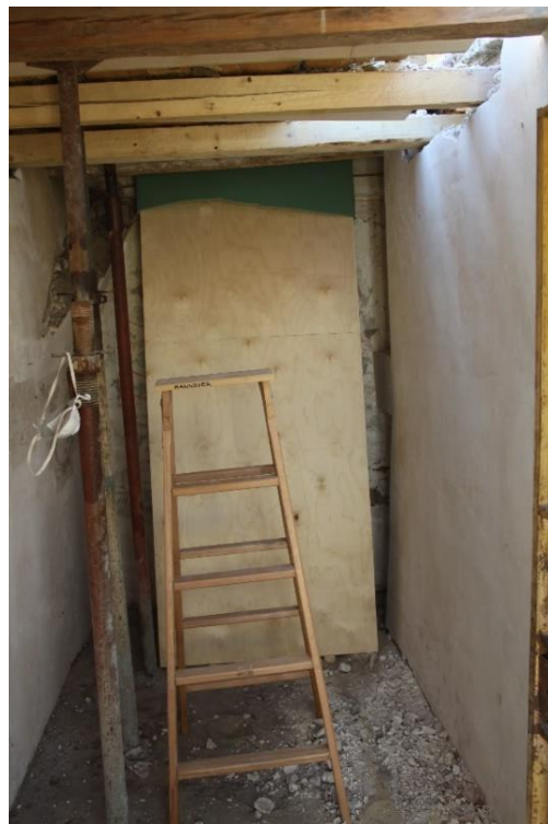
Antechamber (GB33A) (left) and GB33B (right) with protective shields during roof work
